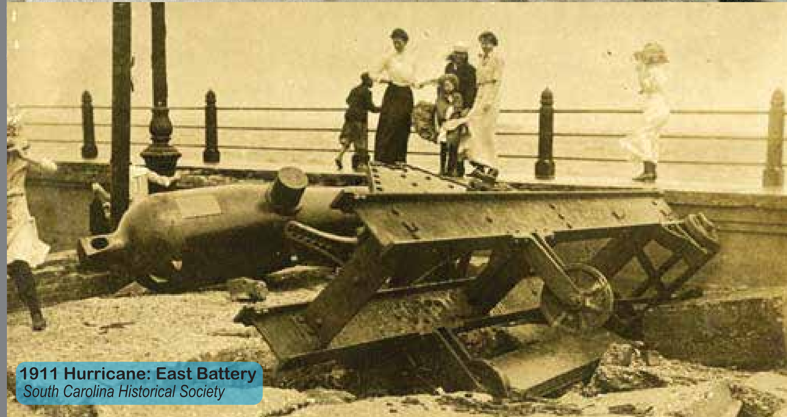
1911 Hurricane: East Battery facing northwest South Carolina Historical Society
